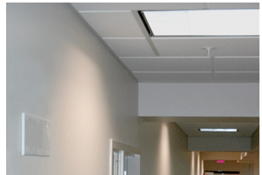
Photo Left: The clean lines of the hallway are preserved utilizing the concealed SentryLight. With nothing to attract attention, and utilizing polycarbonate cover plate and lens housing, maintenance due to vandalism is reduced. A detail is seen above.
